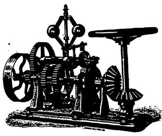
Any deviation from the correct speed, however slight, affects the action of the governor upon the gate, and it quickly brings the speed up or down to its proper point.
