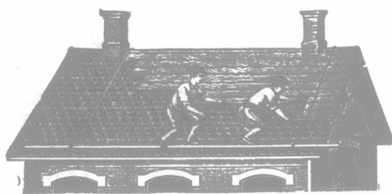
Made from Painted or Galvanized Steel at prices varying from \$2.85 to \$5.10 per 100 square feet, covering measure. This is the most durable covering on the market, and is an ideal covering for Houses, Barns, Stores, Elevators, Churches, etc. Any handy man can lay the "Oshawa" Shingles. A hammer and snips are the only tools required. We are the largest and oldest company of the kind under the British flag, and have covered thousands of the best buildings through Canada, making them
