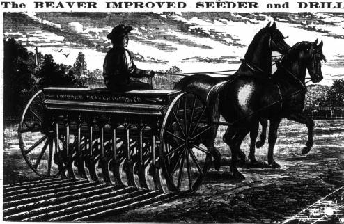
MANUFACTURED ONLY BY THE MASSON MANUFACTURING COMPANY, OSHAWA, ONT. CALIFORIA 12-HORSE DOWN POWER. We know that it has Steel Drag Bars, Steel Frame, Steel Axle and Steel Distributor Rods.
