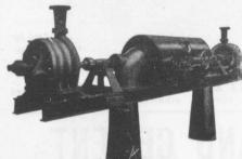
Two Worthington 3-Stage Turbine and McCormack Water Wheels, built for Port Arthur, Ont., Water Works, 1440 gai. per minute against 350 ft. head.
