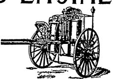
This machine is the most powerful fire fighter. It has two cylinders, 40 gallons capacity each. The combination of chemicals will not freeze, renders material with which it comes in contact non-inflammable, and will not corrode when not in use. For full particulars, write to the Head Office of the Company at Kingston.
