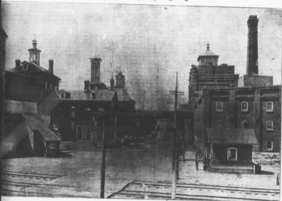
VIEW FROM THE RAILWAY LOOKING NORTH.
