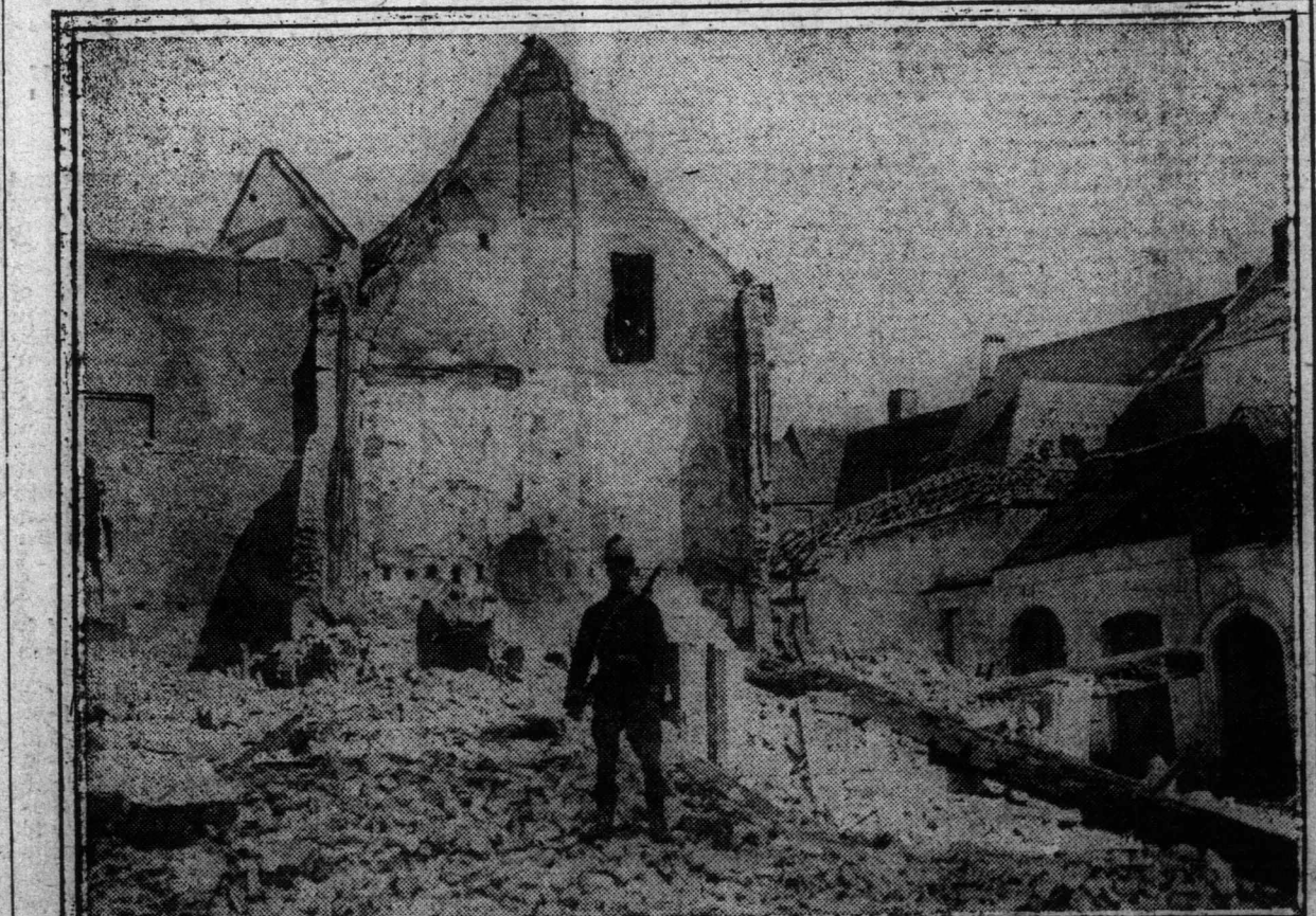
DAMAGED HOUSES IN MALINES On the morning of September 1, seventy-five shells were fired into the unfortified town of Malines, Belgium, by the Germans, the bombardment lasting for one hour and twenty-five minutes. Much damage was done to the Cathedral and other historic buildings, and many rare and priceless pictures were destroyed.
