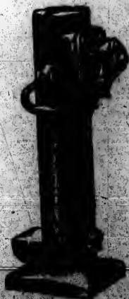
25-ton Foot-Lift Bridge Jack
