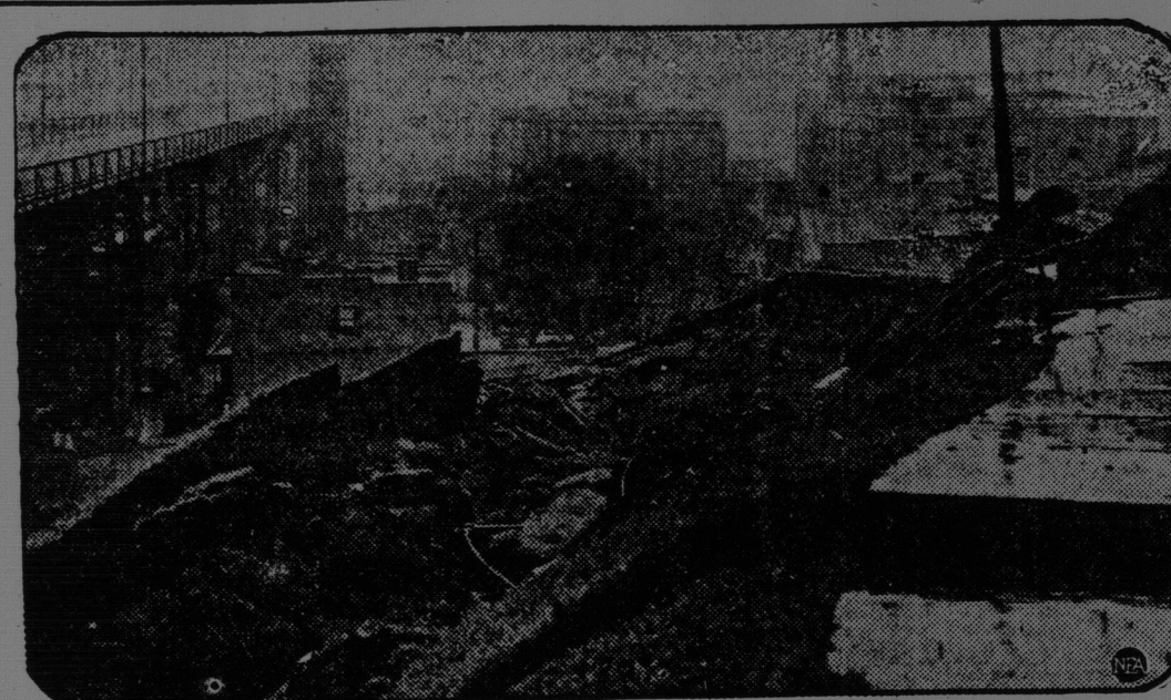
While laborers were at work reinforcing the Chesapeake and Ohio Railroad tunnel at Richmond, Va., it caved in, trapping more than twenty men. Rescuers have been unable to find the bodies of six of those missing. Note the landslide effect in this hillside above the tunnel, and the broken pavement.
