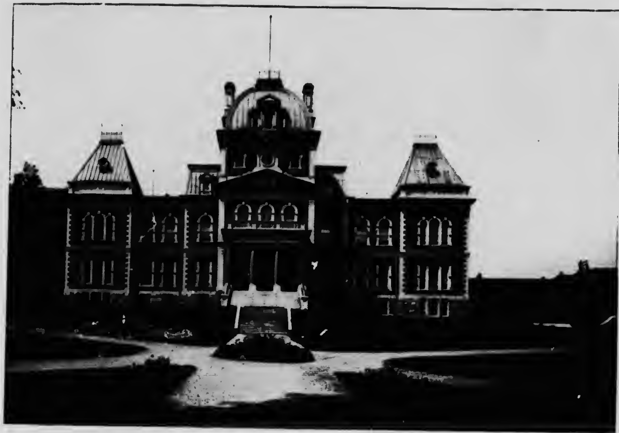
COURT HOUSE AND STRATHCONA SQUARE
