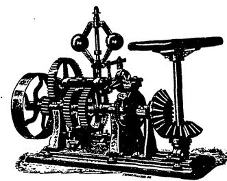
Any deviation from the correct speed, however slight, affects the action of the governor upon the gate, and it quickly brings the speed up or down to its proper point.
