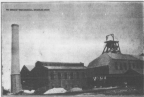
An almost total absence of smoke. A 2,700 h.p. boiler plant in operation. This plant is fired by mechanical stokers and the coal used is "stuck" and crushed splint. The photograph illustrates normal conditions.
