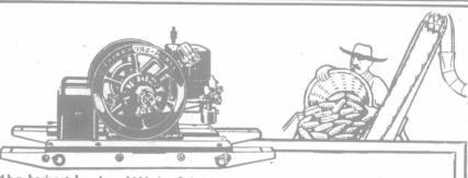
4 h.p. horizontal engine, skidded. Suitable for light work such as grinding, shelling, shearing, running the separator, churn, ètc.
