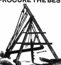
The Whitfield Stump Extractor. The superiority of this machine consists in the rapidity and ease in which it can take out the largest stumps; the ease with which it is operated by man or beast, and the great strength and durability of this machine. It leaves no holes to fill up, nor any stumps or snags in the ground. Send for circular of testimonials and particulars about it before purchasing an inferior machine
