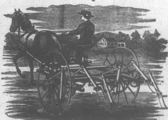
Experience has demonstrated the fact that a good HAY TEDDER that will thoroughly spread long, heavy grass, taking it up from the bottom, tossing it gently into the air, and leaving it upon the ground in a light, fleecy condition, enables the farmer to take advantage of fair weather, and at least twice the quantity of hay can be secured, in better condition, than when allowed to remain in the swath.
