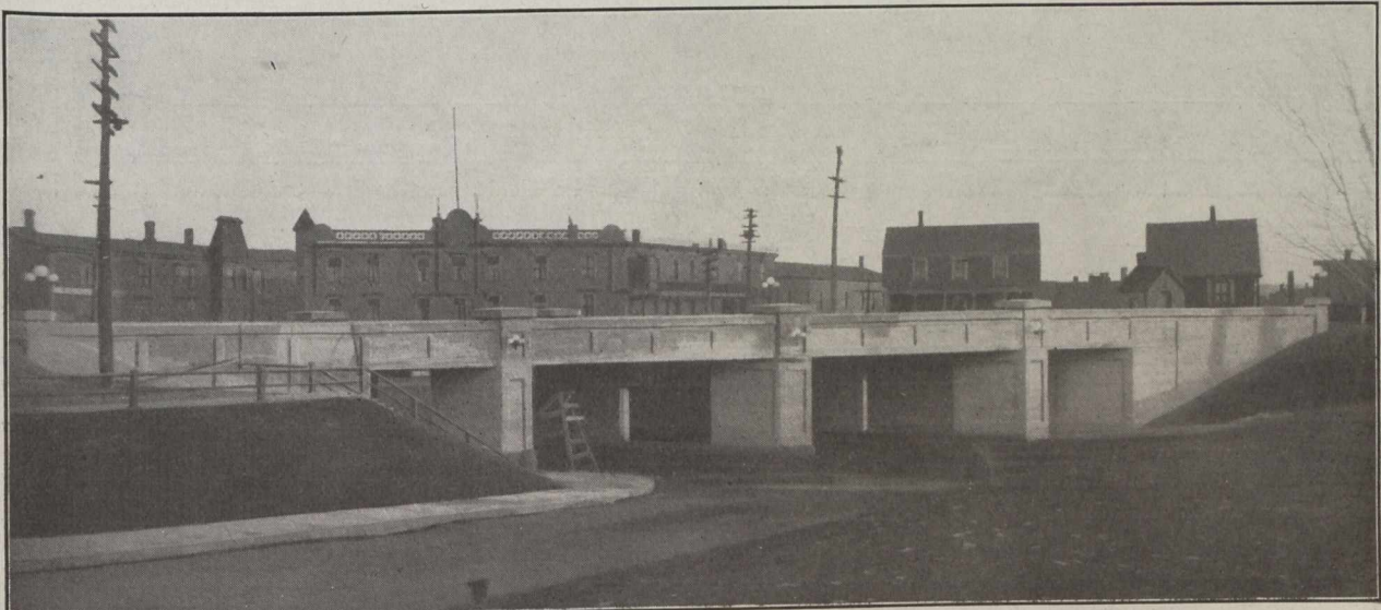
View from Archibald Street of Main Street Subway, Moncton, N.B.
