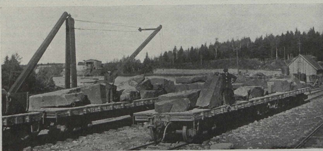
Rock Used in Facing Pier and Breakwater.
