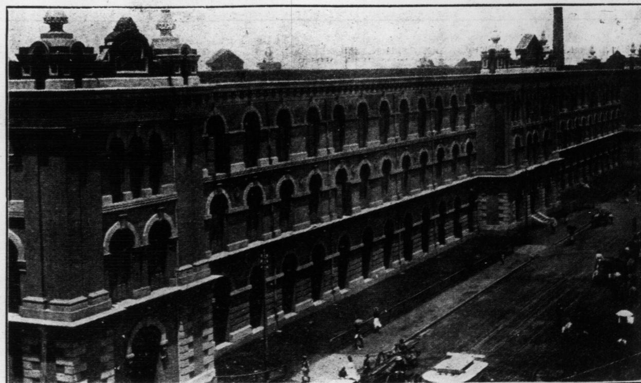
PORT COMMISSIONERS' TEA WAREHOUSE, CALCUTTA.
