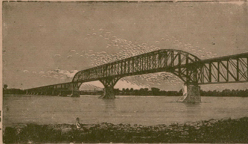
ST. LAWRENCE RIVER BRIDGE, CANADIAN PACIFIC RAILWAY, LACHINE, P. Q.
