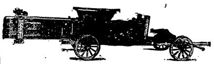
This press has an all steel baling chamber. It has an extremely large feed opening and is a full circle Press. The power works well at any angle so that the machine does not require to be set level. Has gong to tell when dividing board should be inserted.
