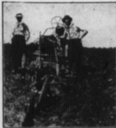
Big Bull Tractor, the largest drive wheel is on the right of the machine. Pulling two 14-inch plows. Built Tractor Co. of Canada, Ltd., Winnipeg.
