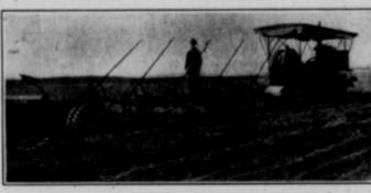
60-H.P. HOLT CATERPILLAR GAS TRACTOR breaking at Namaka Farm, Namaka, Alberta, Canada. Pulling 10 14-inch engine gang and packer.
