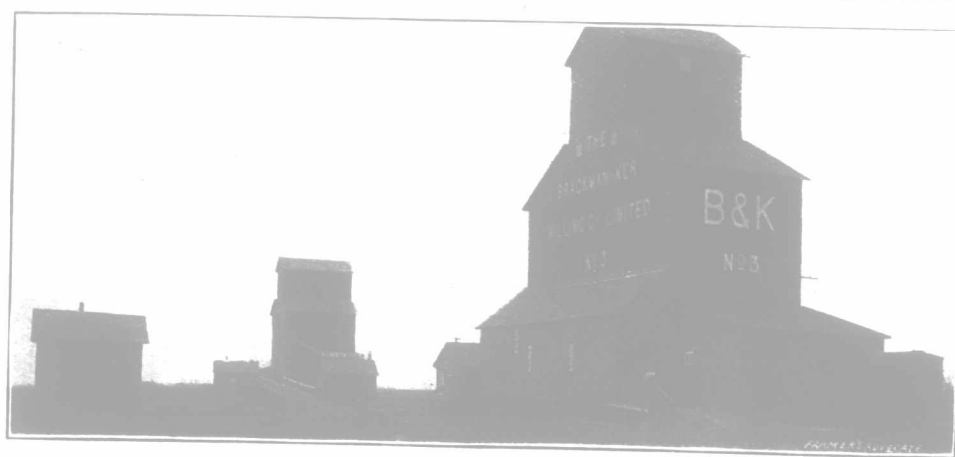
The Elevators at Leduc, Alta.
