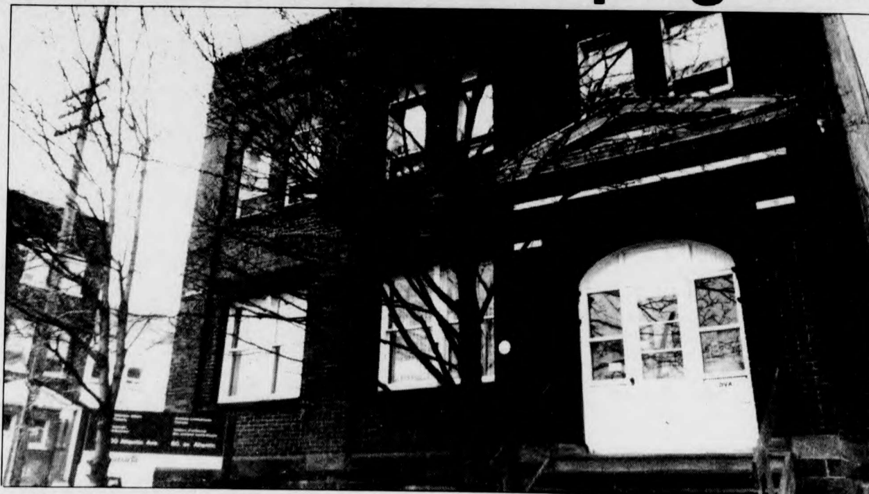
60 ATLANTIC AVENUE: The BCF has proposed that this site be converted to live/work space for artists.
