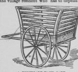
A HOMEMADE HAND CART. elbarrow, or some such arrange as this to move his small crops and other stores. The sides and ends fit tightly into iron sockets, and, for stability, lock to-gether at the corners when in place, as shown in the engraving. Any one handy with tools can construct a very serviceable rig of this sort, the only necessary adjuncts being a pair of wheels, which are often at hand, from some broken or worn-out wagon, sulky, or other light vehicle.—Amorican Arginaltunic
