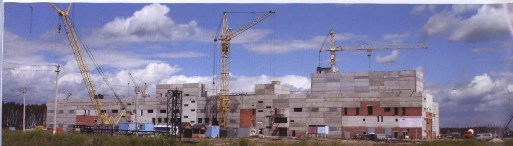
Second main destruction building, Shchuch'ye chemical weapons destruction facility
