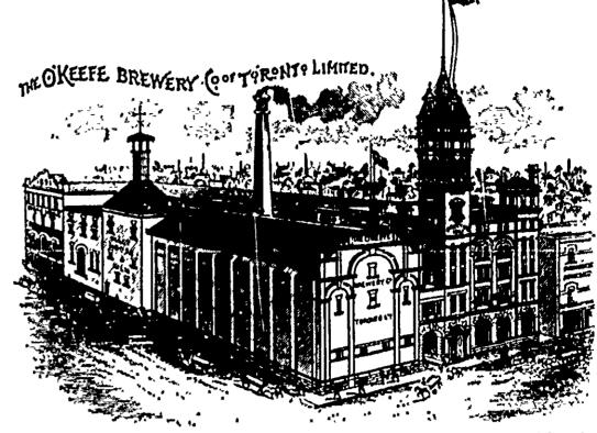
ONE OF THE MOST COMPLETE BREWERIES ON THE CONTINENT. Capacity, 163,000 barrels annually Kquipted with the root modern plant, including a De La Vergou Refrigerating Machine, 75 H.P., with Wate Tower in connection; a 75 H.P., Electric Dyramo for lighting Brewery and running several Motors; a large Water Filter toapacity 2,000 gallons per hour, through water, after passing, is absolutely pure and is used in all browings. Our improved facilities enable us to guarant so our products.
