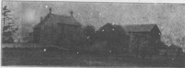
Electric Energy is Used in Both House and Outbuildings. This is one of the seven farmsteads near Waterloo enjoying the benefits of Hydro-Electric connections; the home of Mr. Eldon Hallman.
