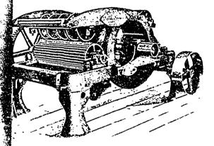
movable Bridge to Permit Saws to be Withdrawn from Mandrel. Feed Pulley 's Readily Removed.
