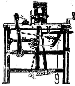
The above Cu; No. 1 shows some very important changes that have lately been made, which makes the machines for less complicated for new beginners to operate. Cut No. 2 shows this machine with a circular saw upon it ready for operation.
