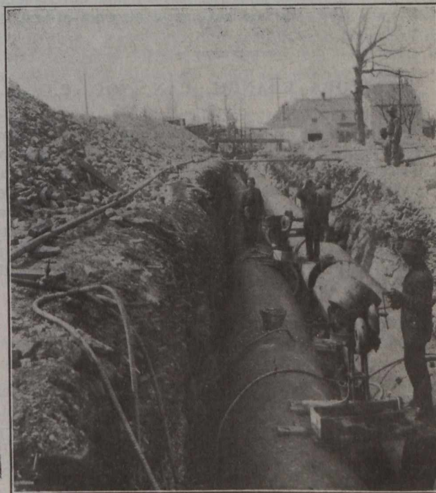
Fig. No. 7.—Riveting Pipe in Trench
