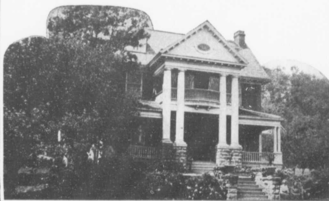
A Fourth Ave. West Residence
