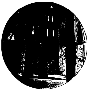
INTERIOR OF CANTERBURY CATHEDRAL.
