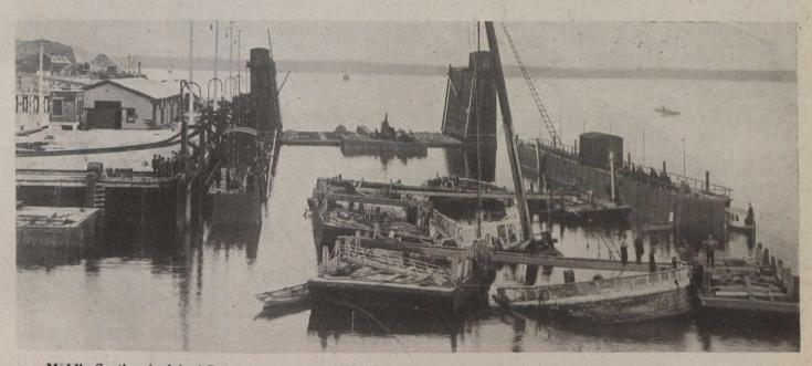
Middle Section (only) of Dock Submerged. Wrecked Vessel "Delhi" Being Lightered onto Submerged Section. One End Section, Not Submerged, in Background.
