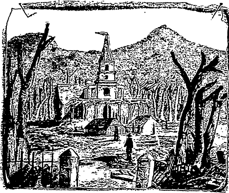
MAURITIUS CATHEDRAL AFTER THE HURRICANE.
