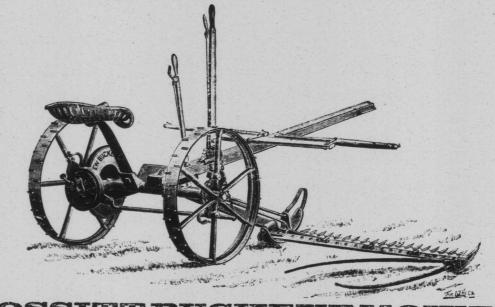
improved for the season of 1893. The removal of the Leading wheel and the light Malleable inside shoe allow perfect freedom of tilt and with the improvement in the shifting gear constitute it the lightest draft and most easily handled as well as the most durable and satisfactory Mower in the Market.
