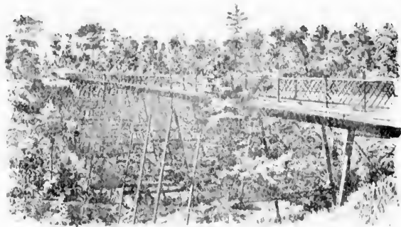
BRIDGE SPANNING THE RAVINE.
