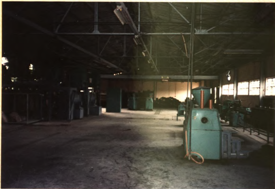
No. 19. View of a small portion of the woodworking plant. Note concrete floor and steel building construction.
