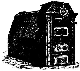
This Boiler is built with sheet steel case or for brick easing as desired.
