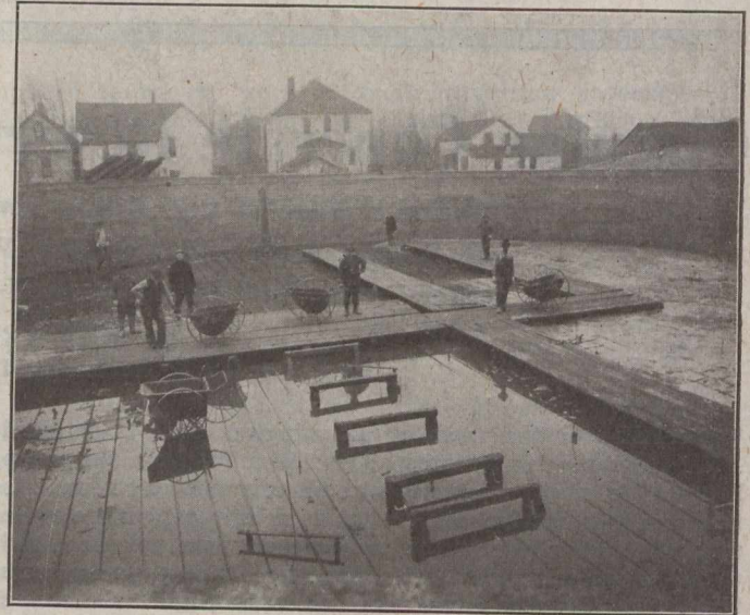
POURING FLOOR FOR RESERVOIR
