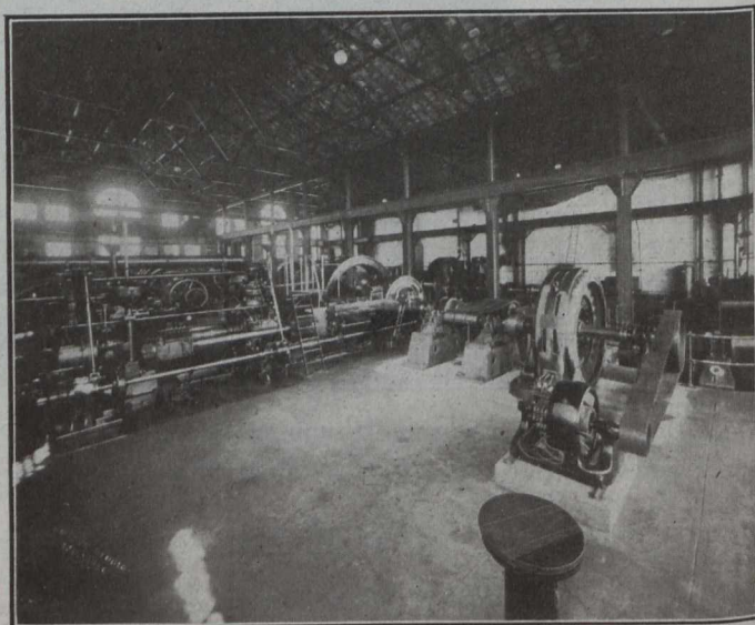
High Speed Generator Unit With Silent Chain Drive. Photo, July 26th, 1917
