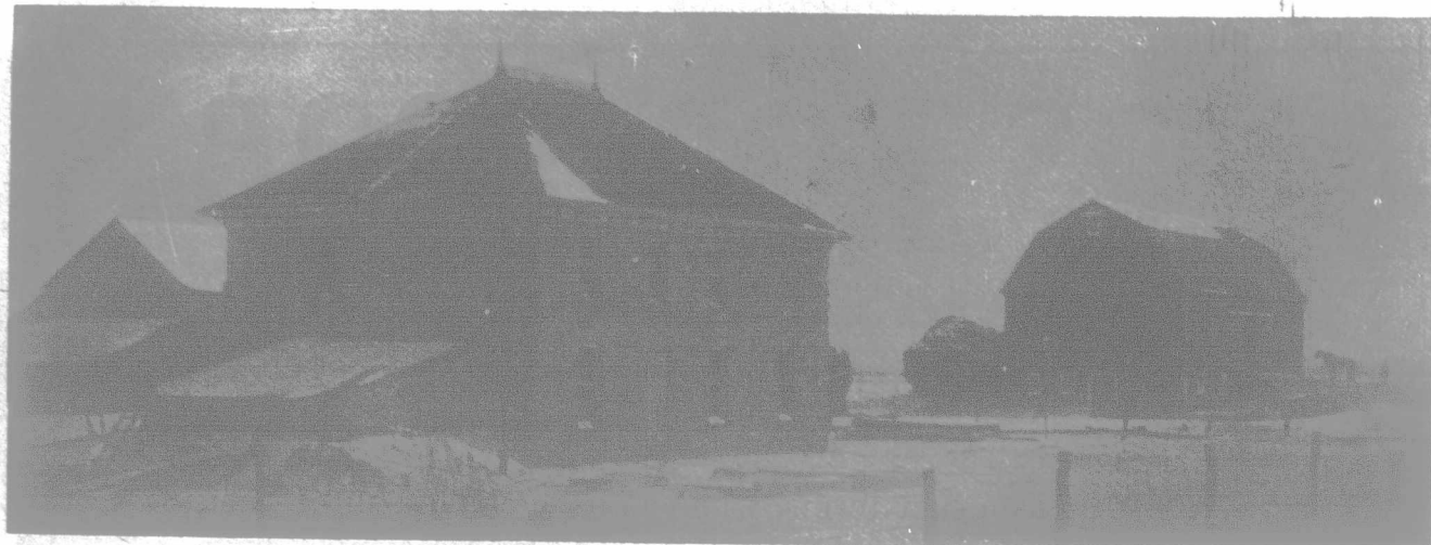
HOUSE AND BARN OF MR. J. E. REAVELY, AT MARSHVILLE, ONT. (Size of house, 28x40x22 high. Size of barn walls, 40x80x10.)
