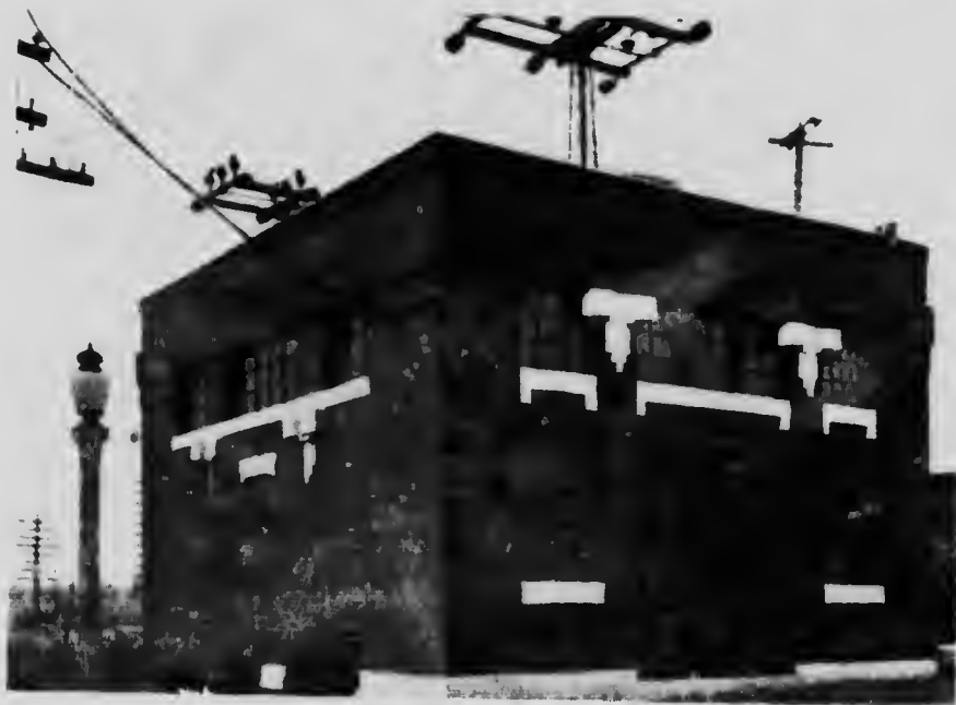
Fig. 1,945. An Automatic Substation on the Great Lakes.
