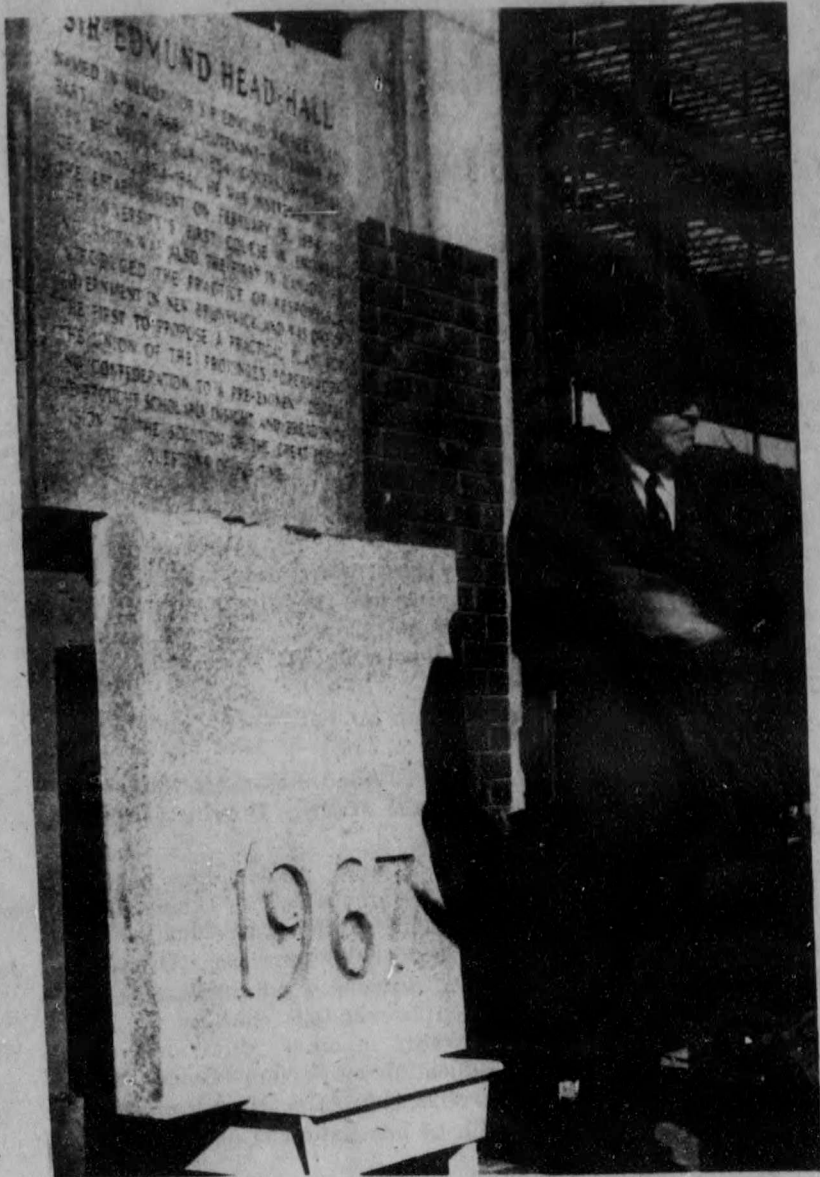
Dr. A. Foster Baird, professor emeritus of electrical engineering at UNB and member of the University's faculty from 1916 until his retirement in 1951, headed the list of cornerstone-laying guests at the new Engineering Building. The cornerstone was laid for the building's three million dollar extension, expected to be completed late in 1967.
