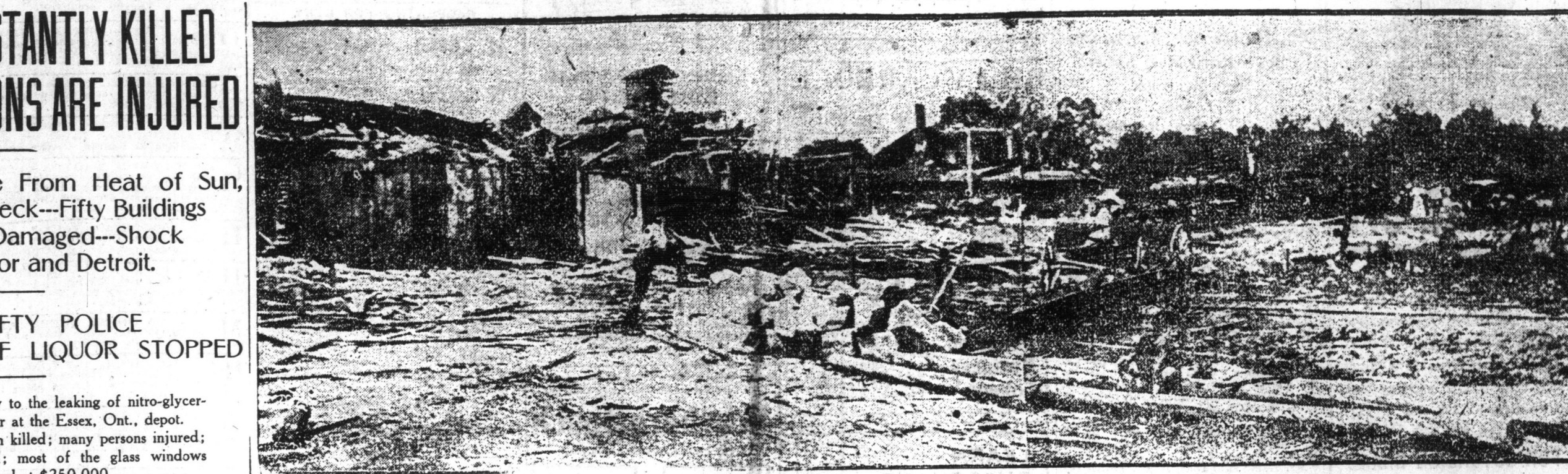
THE EXPLOSION AT ESSEX—Scene in the Railway Yards, Showing the Wrecked Buildings in the Vicinity.
