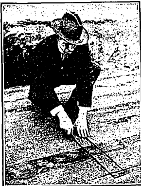
Photograph shows the first step of the test cut, to which every Barrett Specification Roof guaranteed by us is subjected.
