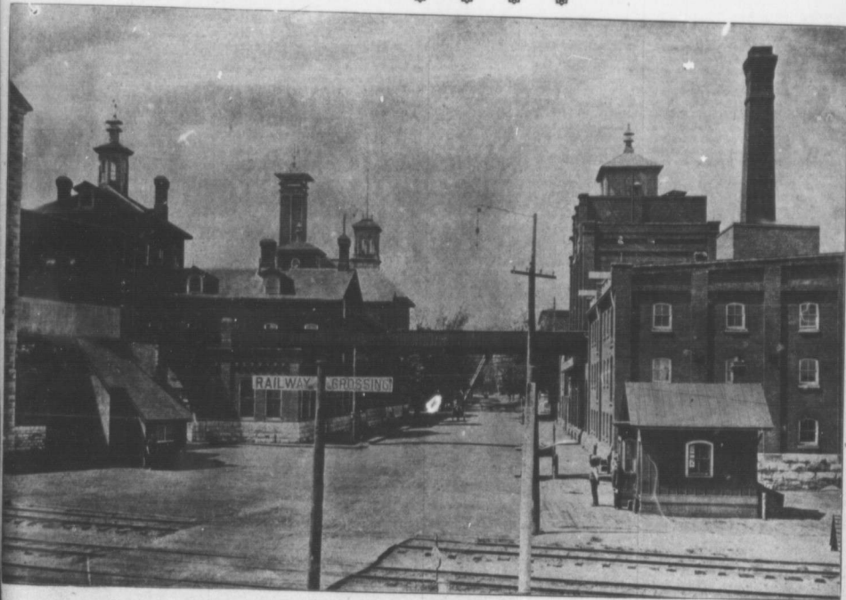
VIEW FROM THE RAILWAY LOOKING NORTH.
