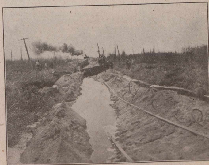
BUILDING THE C.P.R. THROUGH A SWAMP
