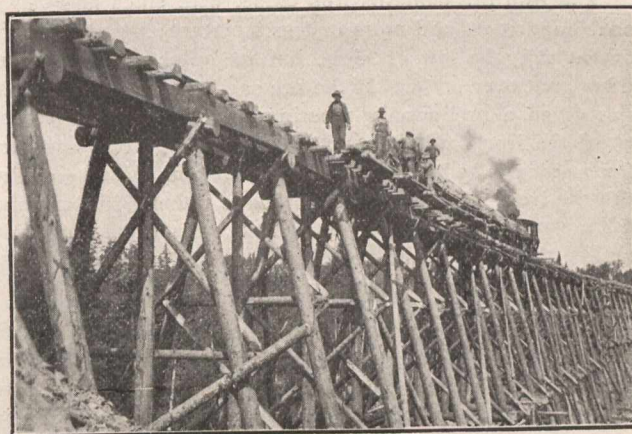
Mullin's Brook Trestle just before the Collapse.
