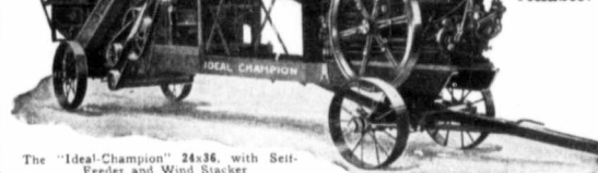
The "Ideal-Champion" 24x36, with Self-Feeder and Wind Stacker
